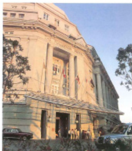
Hotel entrance with glass and steel canopy
