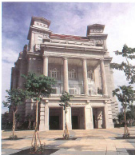
Exterior facade in Singapore plaster finish with grand Doric columns
