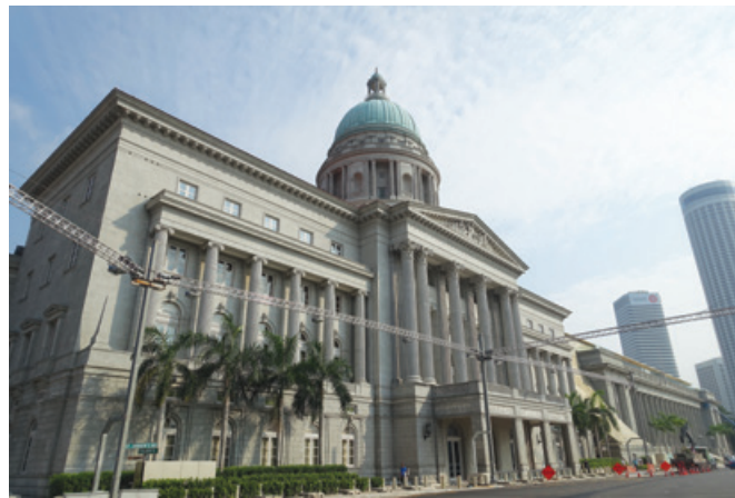
Former Supreme Court and City Hall adapted and integrated as the new National Gallery Singapore
