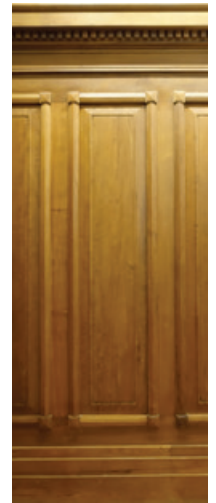
Careful treatment of original timber
