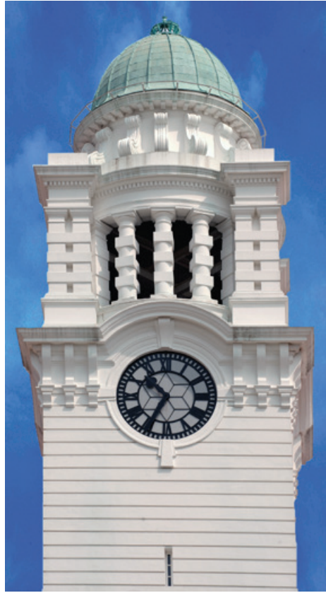
Crown modelled after original reinstated above copper dome
