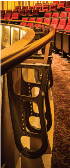
Old chair frames used as balustrades at Victoria Theatre
