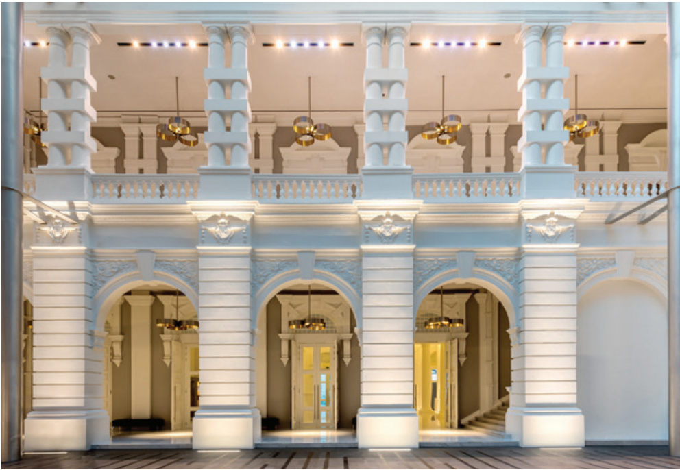
Victoria Concert Hall's atrium façade
