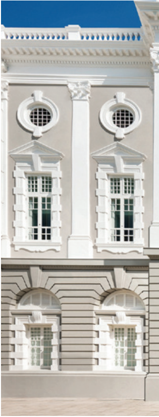
Crisply restored plaster-works on the façade
