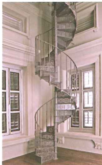
Restored spiral staircase leading to roof
